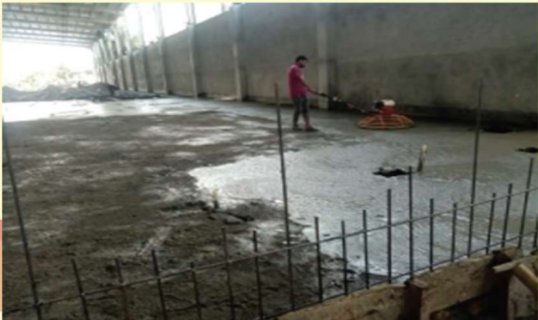
Figure: Floor hardening work, Rising Industries Ltd., Manikganj.
