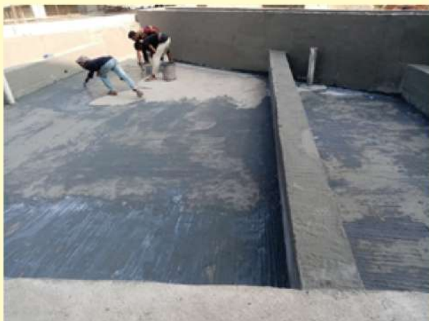
Figure: Cementitious coating work at Villa Golpogriho, Kanchon.
