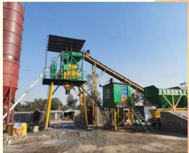
Figure: LGD Road Project, Volagang, Sylhet.
