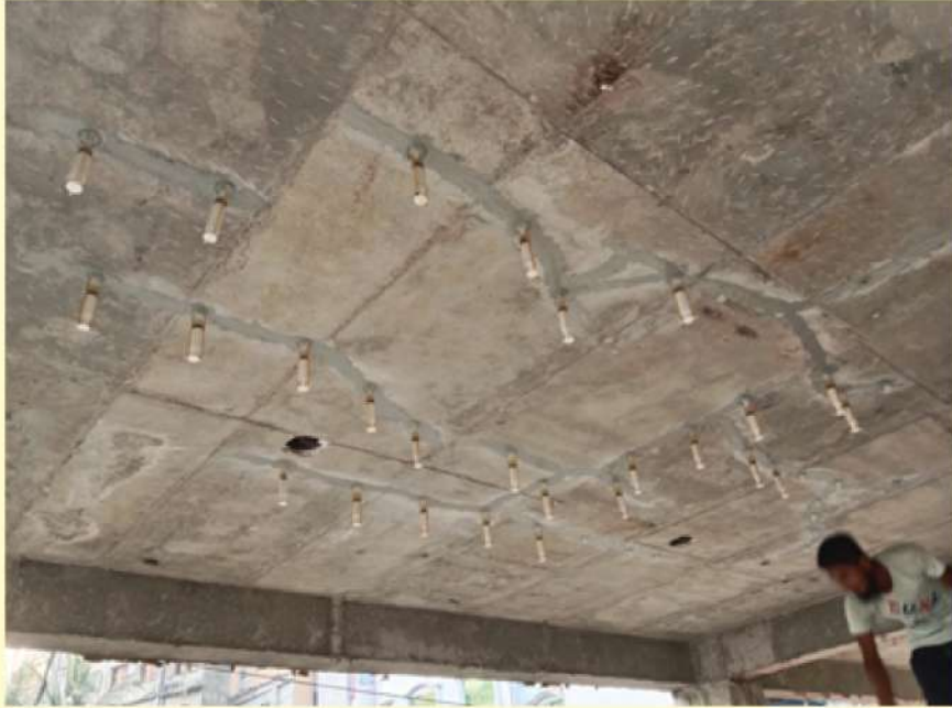
Figure: Epoxy injection work at Oporijita School, Narayanganj.
