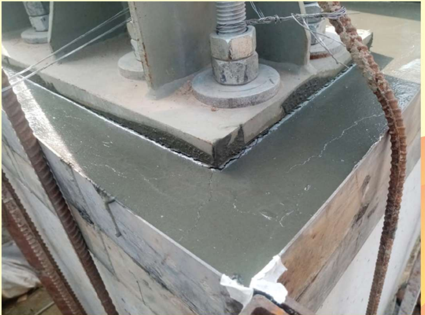
Figure: Non-shrink grouting work at Healthcare Formulations Ltd., Sreepur, Gazipur.
