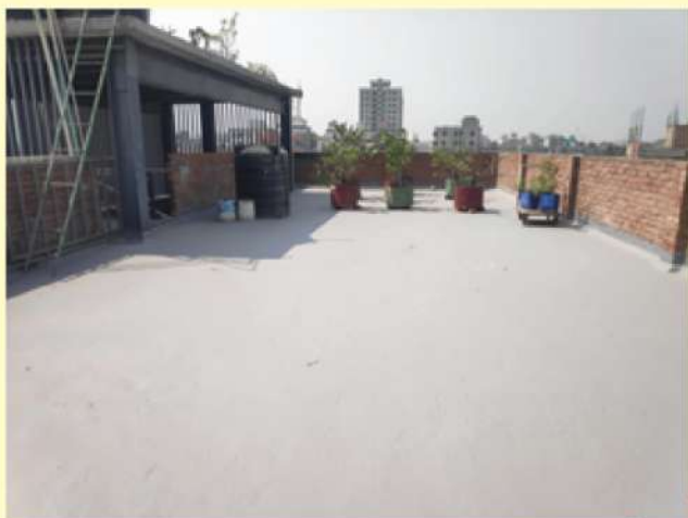
Figure: Open waterproof rooftop coat, Masco industries, Gazipura-27.
