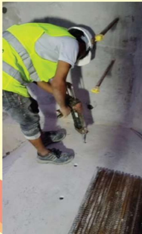
Figure: Rebar anchoring at Sheikh Shiraj's House, Uttara.
