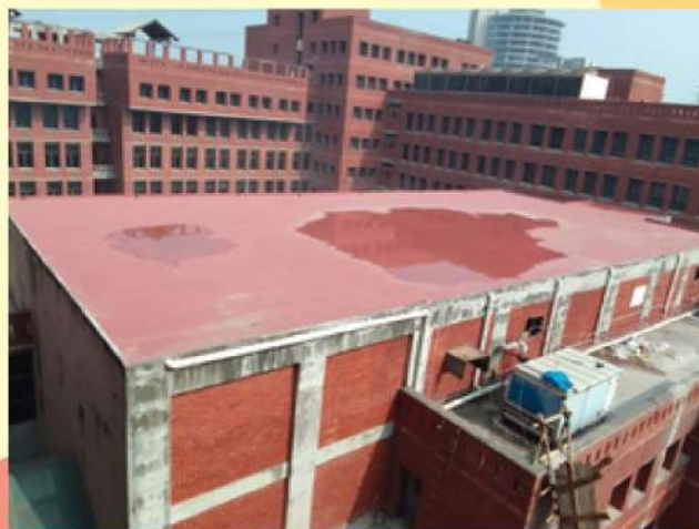
Figure: Open waterproof rooftop coat, East West University, Aftab Nagar.
